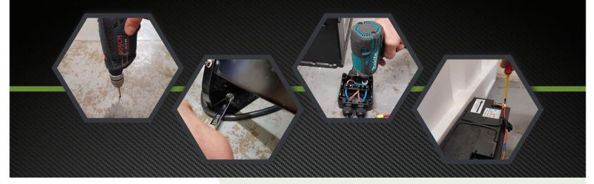
Tighten the PowerUPHD into position, taking care to ensure that the PowerUPHD is level, square and is not being distorted by over tightening or fixing to uneven surfaces. Check once again that the PowerUPHD is free from any obstruction and fix the Positive and Negative power cables to your battery.
